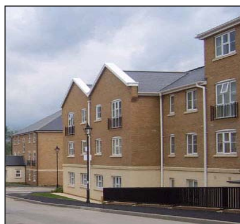
Affordable housing at Elizabeth Jennings Way
